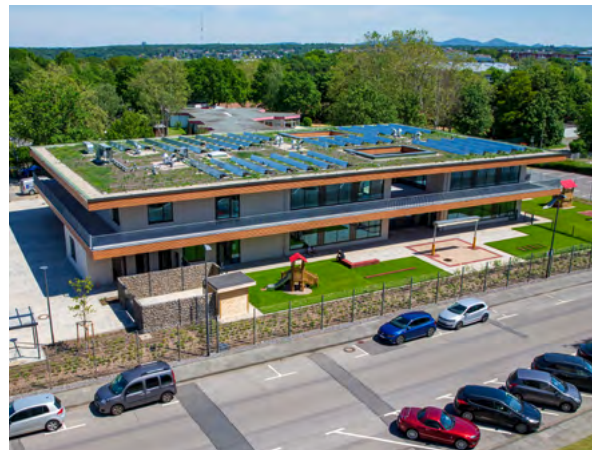
Figure 15: Photovoltaic system on the roof of a Bundeswehr building; Source: Bundeswehr/Marcus Rott
